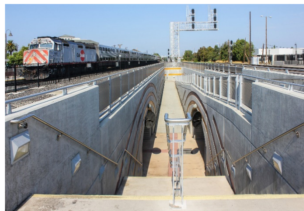
ABC Category 3 Example: Santa Clara Caltrain Pedestrian undercrossing. VTA constructed a tunnel under Caltrain and future BART tracks at the Santa Clara Caltrain Station. Photo: VTA.
