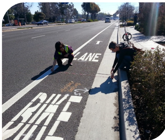
City of Sunnyvale worked with Caltrans to install bicycle lanes on El Camino Real as part of a repaving project. Photo: VTA
