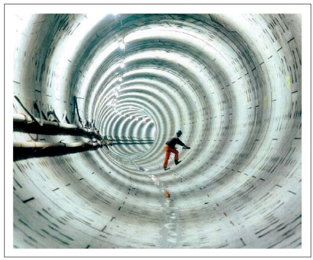
Figure 6-24: Example of Segmental Concrete Lining Units and Rings
