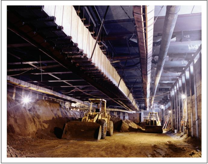
Figure 6-15: Temporary Utility Support in an Excavation
