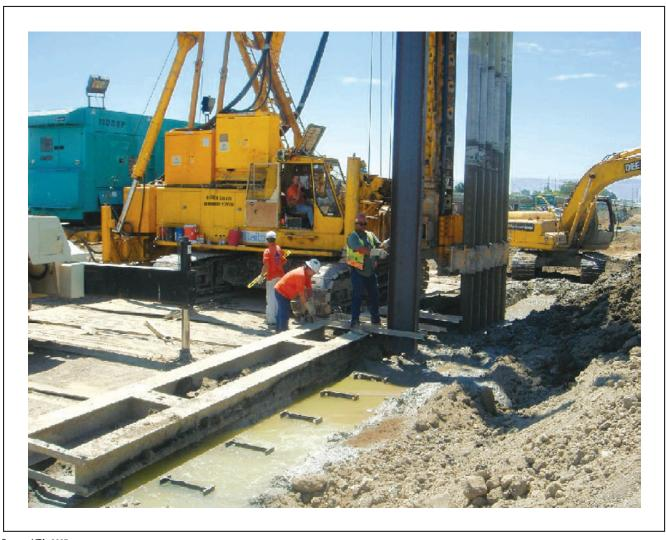
Figure 6-17: Deep Soil Mix and Steel Soldier Pipes
