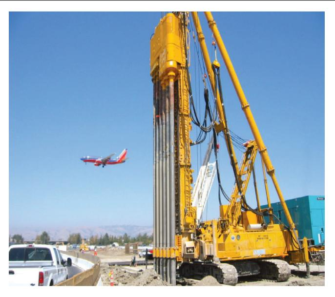
Figure 6-16: Deep Soil Mix and Auger Rig Installation
