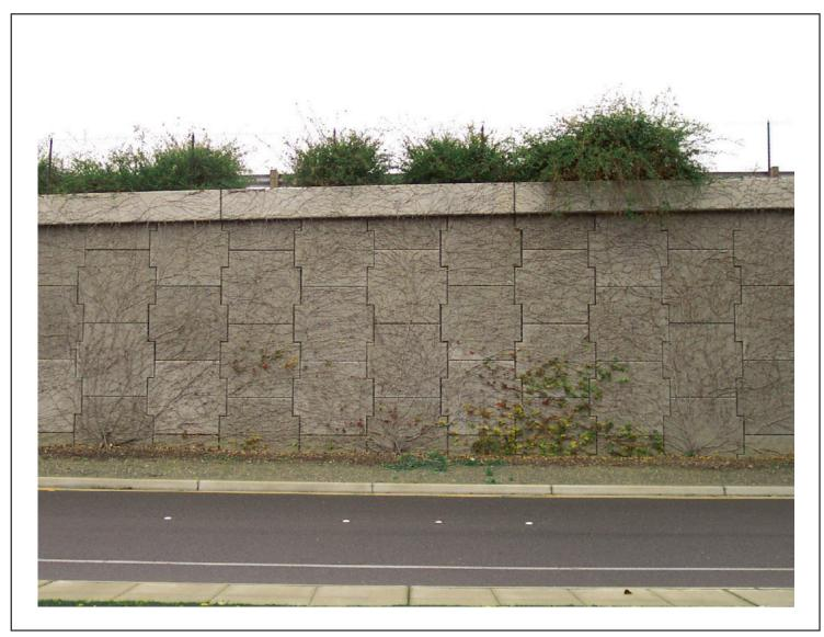
Figure 6-5: Mechanically Stabilized Earth Wall
