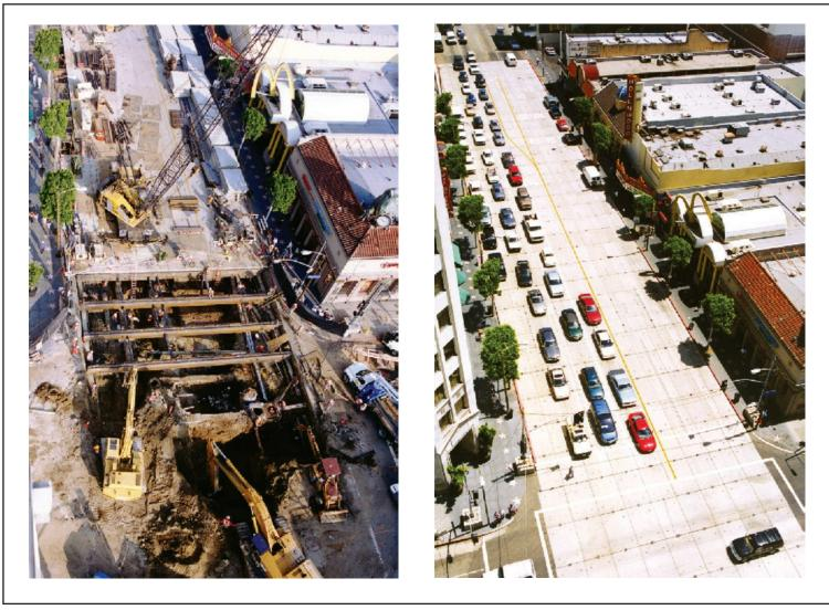
Figure 6-13: Temporary Deck Installation
