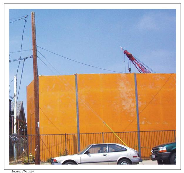
Figure 6-48: Example of a Temporary Noise Barrier
