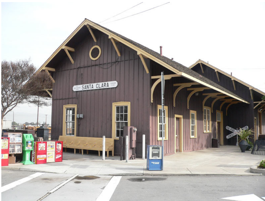
Figure 7-20: Historic Santa Clara Caltrain Station
