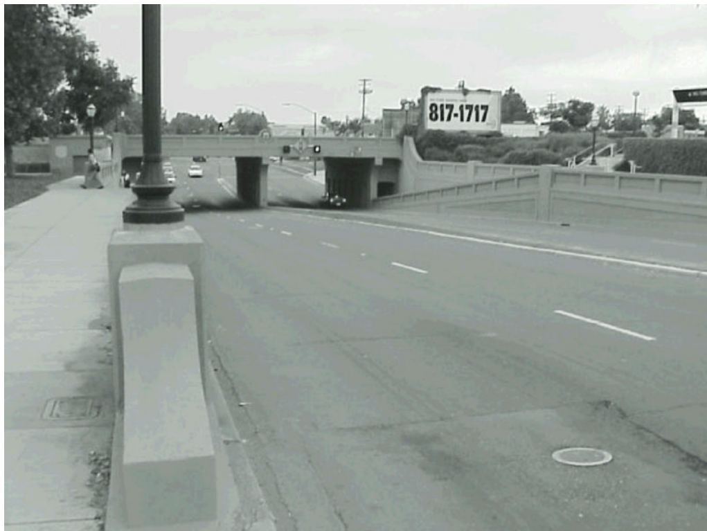
Figure 7-16: Santa Clara Underpass
