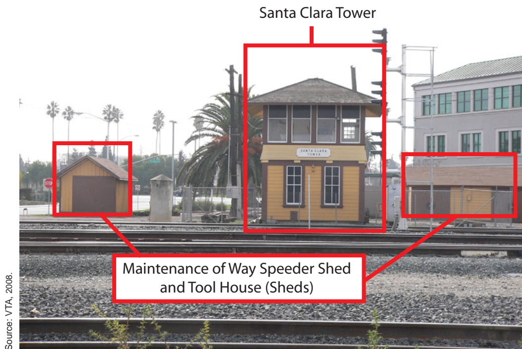
Figure 7-21: Santa Clara Tower and Sheds
