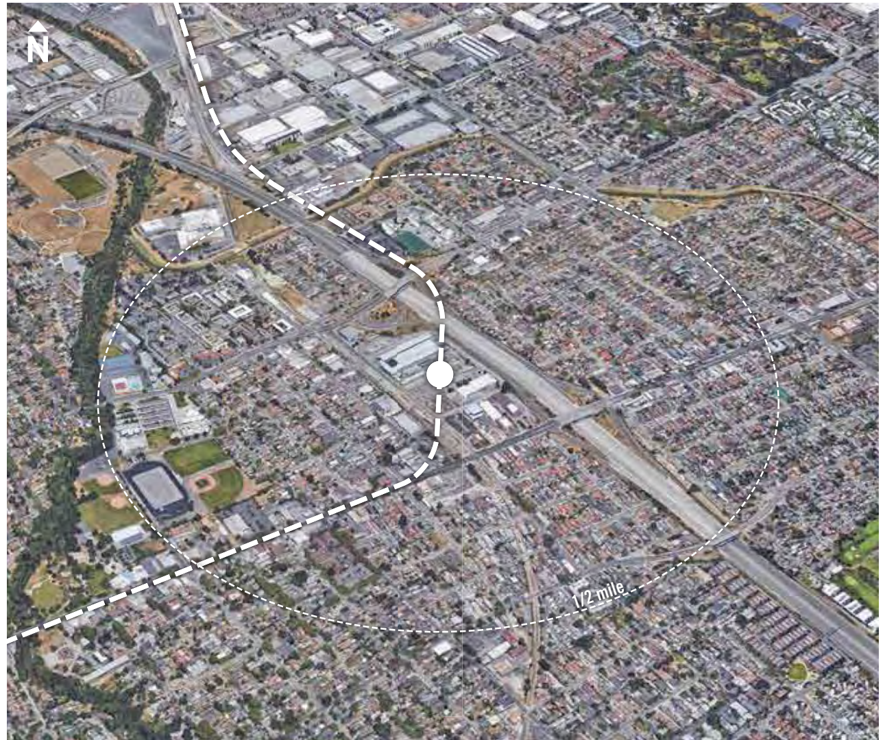
28th Street Station Aerial Overview
