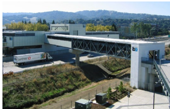
West Dublin/Pleasanton Bridge
