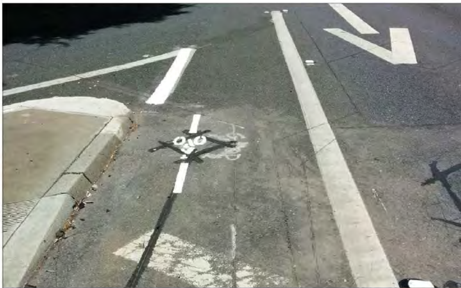
b. View of a bike detector embedded in a bike slot. The purpose of a bike detector is to detect a bicyclist approaching an intersection and communicate with the traffic signal cabinet to provide enough time for cyclists to safely cross an intersection.
