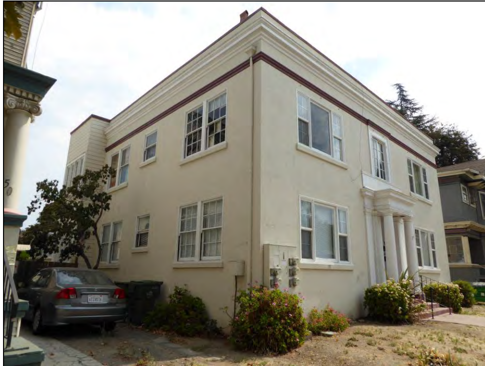
Photograph 3: North and west sides of Colonial Revival building; facing northeast, September 14, 2015.
