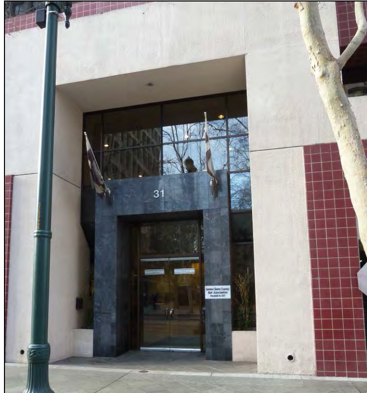
Photograph 2. Main entrance, camera facing west, January 15, 2015.
