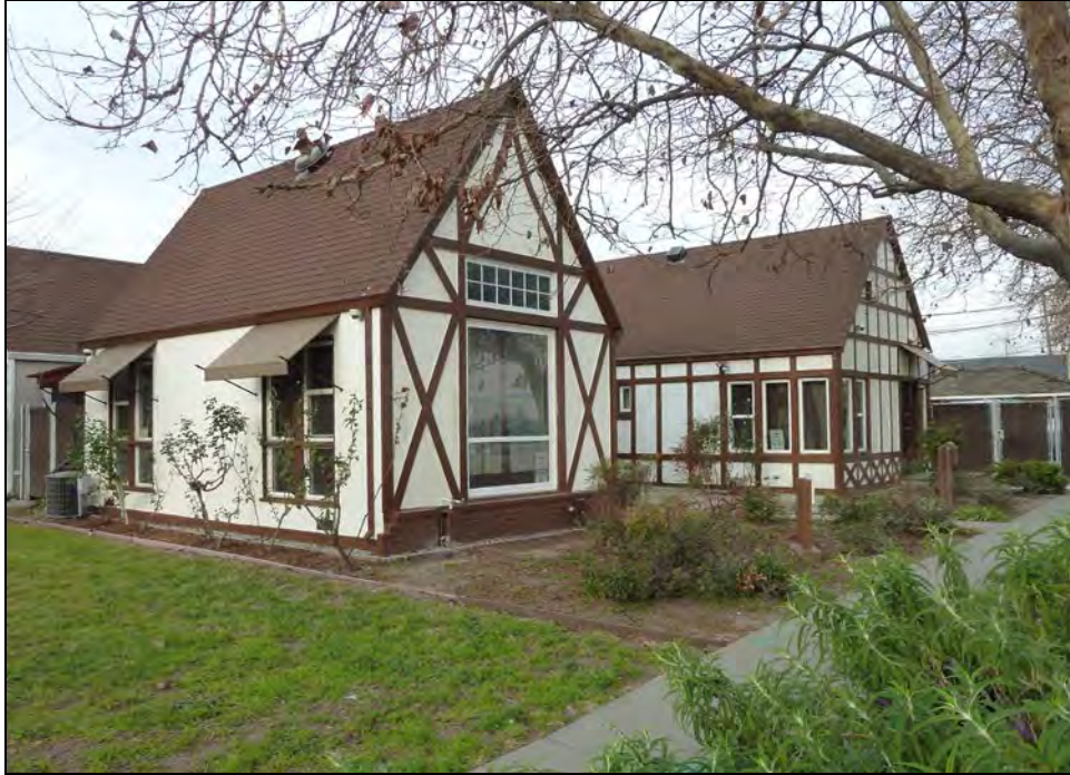
Photograph 2: South and east sides, camera facing northwest, January 16, 2015.
