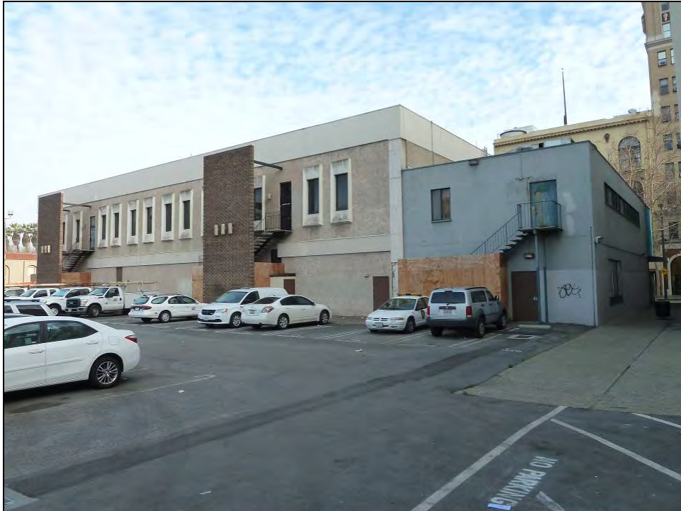
Photograph 3. Showing rear of buildings, camera facing northeast, January 15, 2015.
