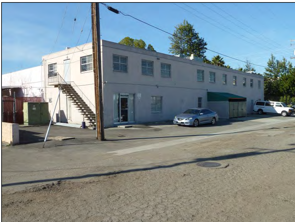
Photograph 3. East end of building, camera facing northwest, January 14, 2015.
