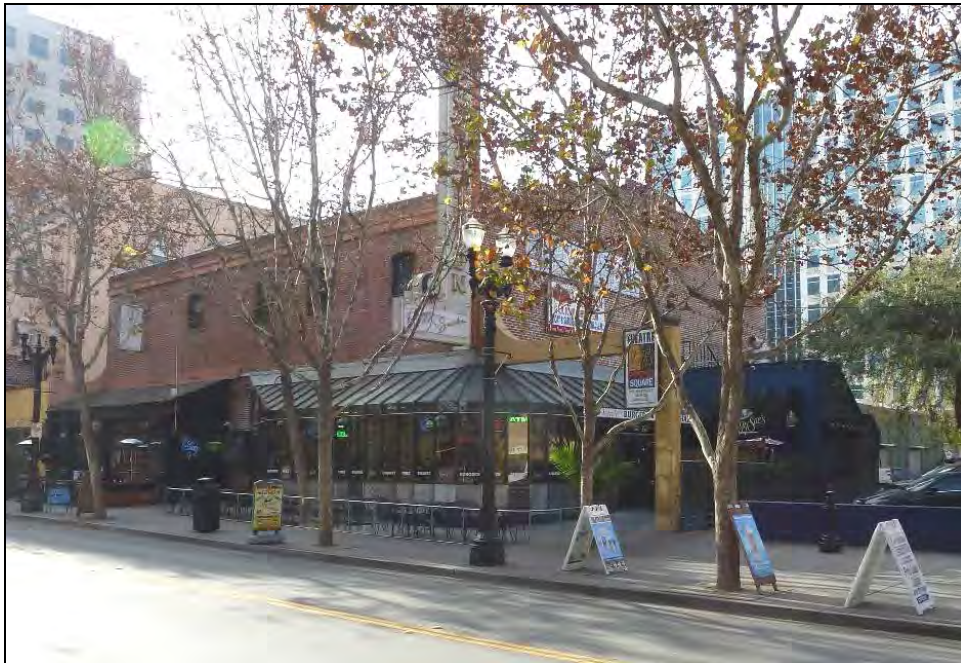
Photograph 2. Old Mill Building, 25-29 N. San Pedro Street; camera facing south, January 15, 2015.
