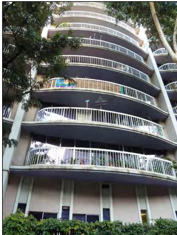
Photograph 3. Balconies, facing southeast, January 14, 2015.
