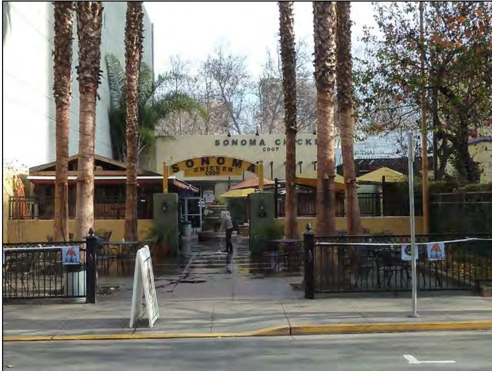
Photograph 2. Rear of building fronting North San Pedro Street; Camera facing east, January 15, 2015.
