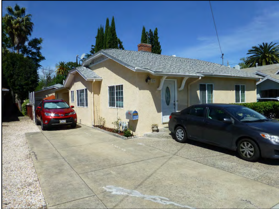
Photograph 2: South and east sides, camera facing northwest, April 20, 2016.
