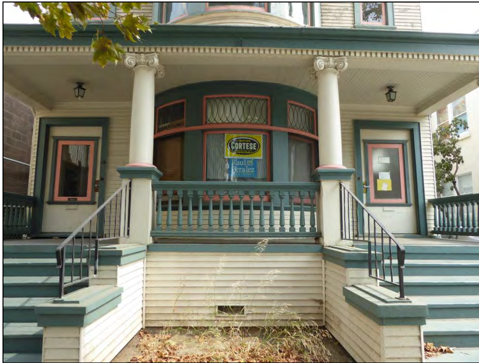
Photograph 2: Detail view of porch, facing northeast, September 14, 2015.
