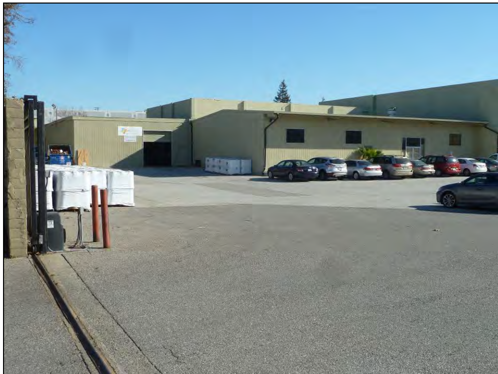
Photograph 3. Sections F, G, and H, camera facing east, January 14, 2015.
