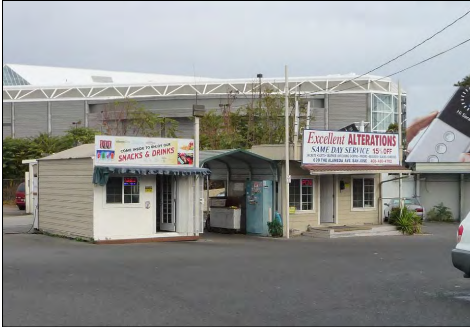
Photograph 2: Building 1 at right (699 The Alameda), Building 2 at left with modern metal carport in between; facing east, November 19, 2013.
