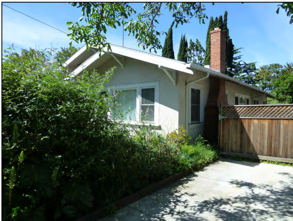
Photograph 3: North and east sides; facing west, April 20, 2016.
