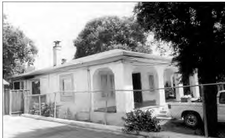
Rear house, view from SW
