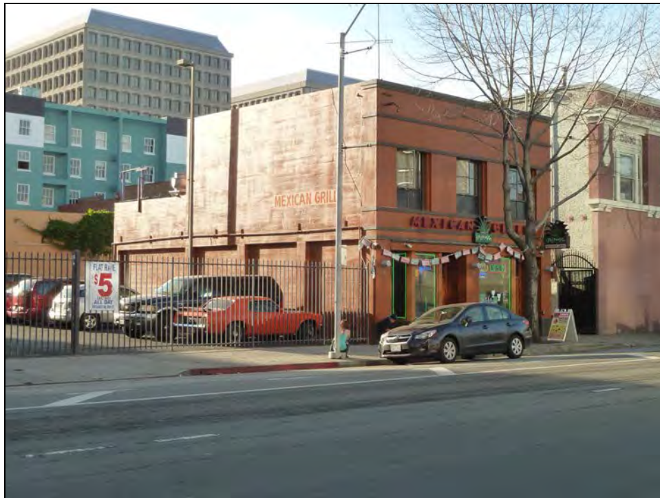
Photograph 2. Camera facing northwest, January 14, 2015.
