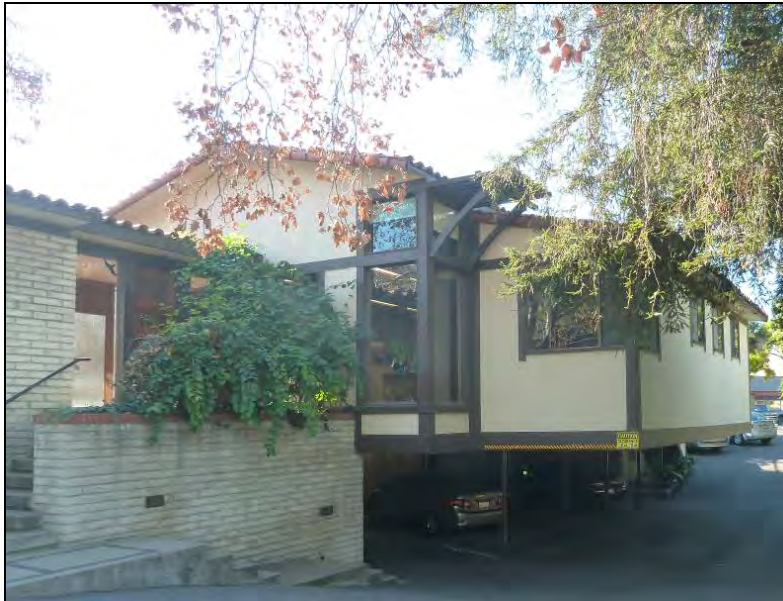
Photograph 2: 945 W. Julian Street, facing southwest, December 4, 2013.
