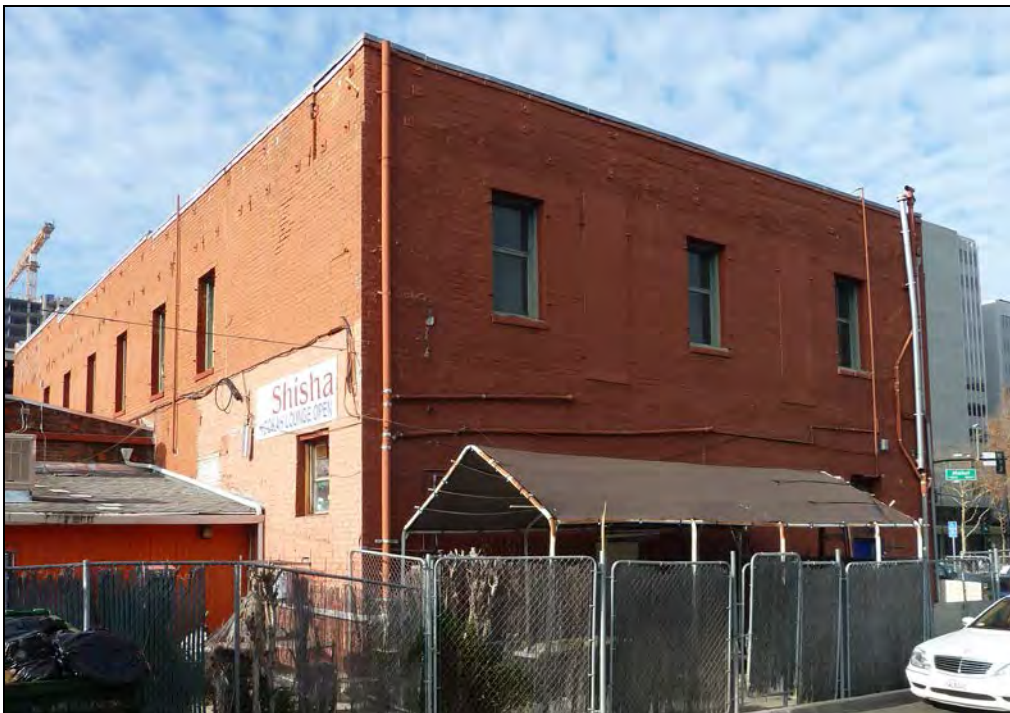
Photograph 2. Rear of building, camera facing northwest, January 15, 2014.
