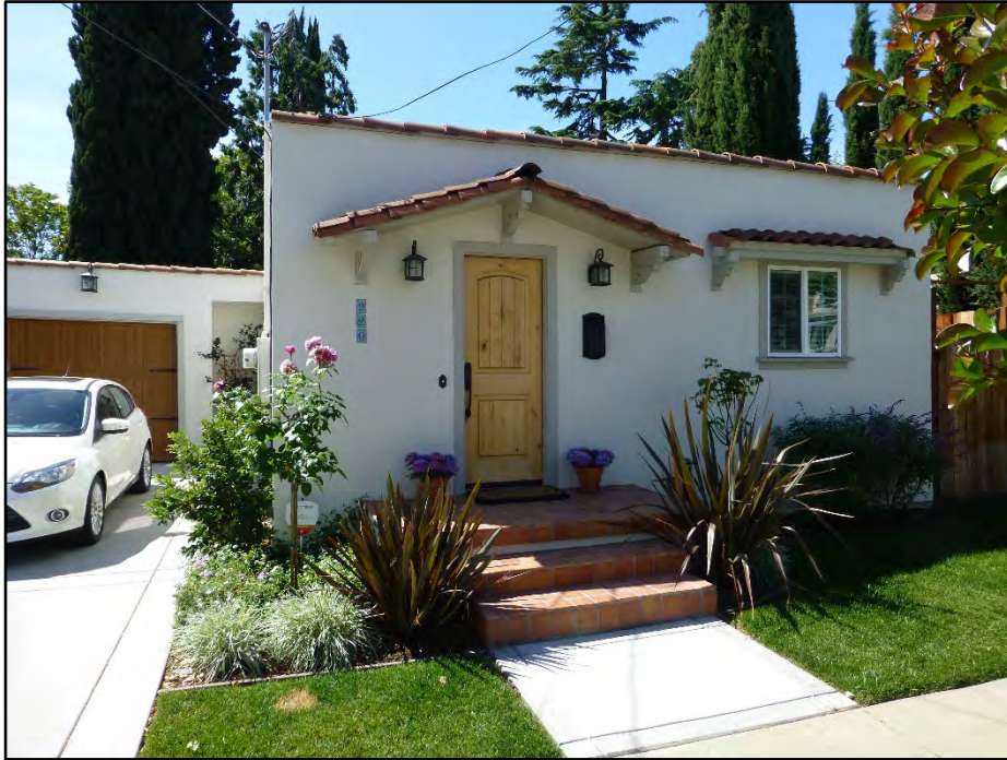
Photograph 2: 920 West Julian Street, camera facing south, April 20, 2016.
