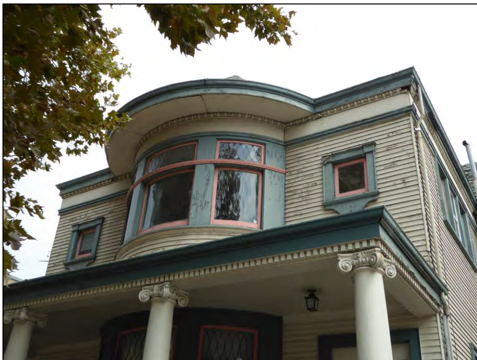
Photograph 3: Detail view of the second-floor of the façade; facing northeast, September 14, 2015.
