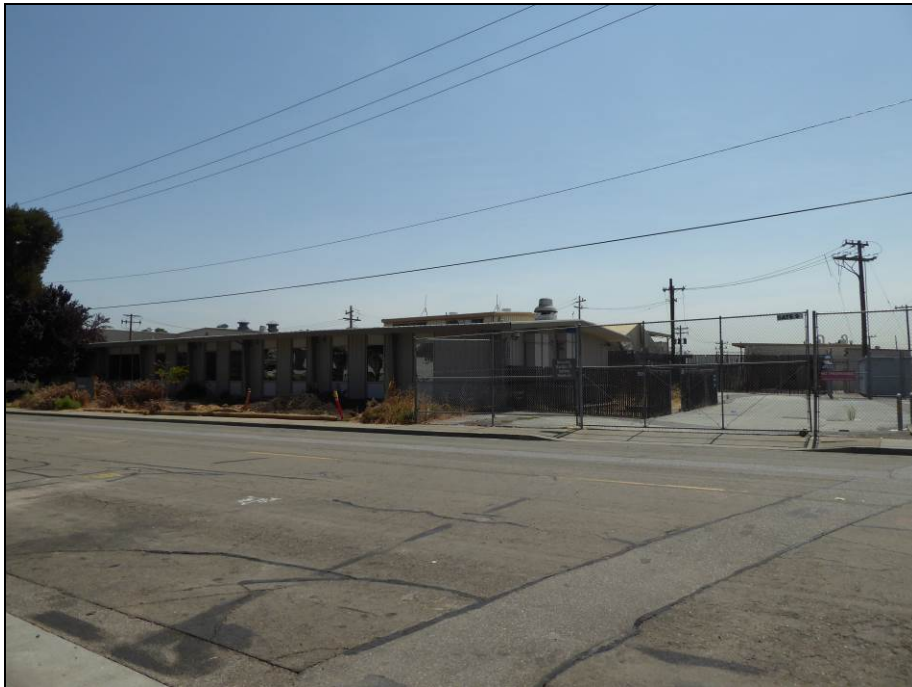
Photograph 3: Former FMC Corporation Office (Engineering Systems Divisions, 328 Brokaw Road) on APN 230-46-069; camera facing northeast, July 26, 2016.
