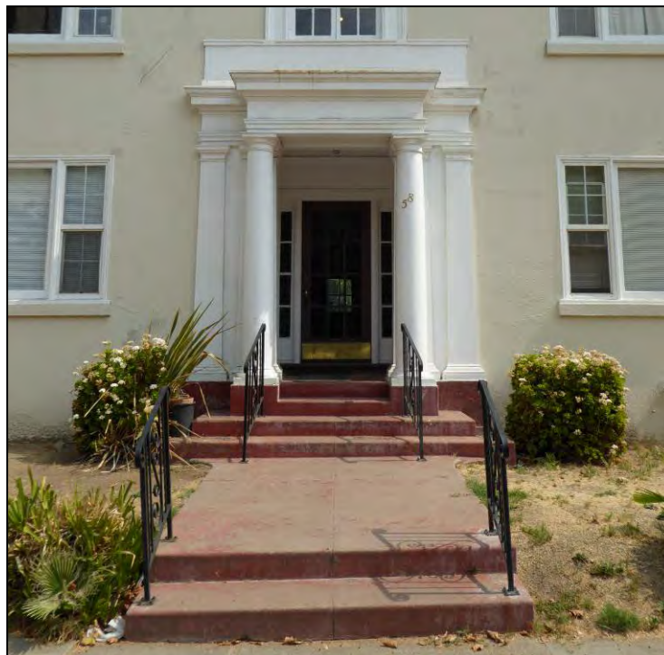
Photograph 4: Detail of main; facing east, September 14, 2015.
