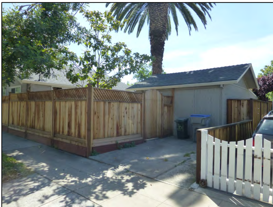
Photograph 3: Garage; facing southeast, April 20, 2016.
