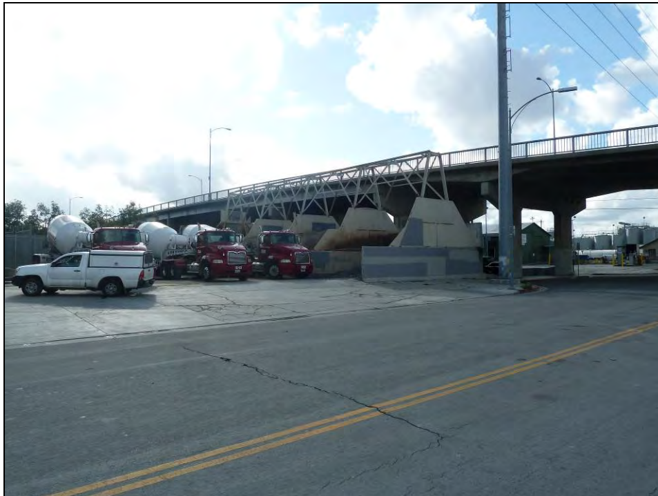
Photograph 2: Showing materials storage structure, camera facing northwest, March 26, 2014.
