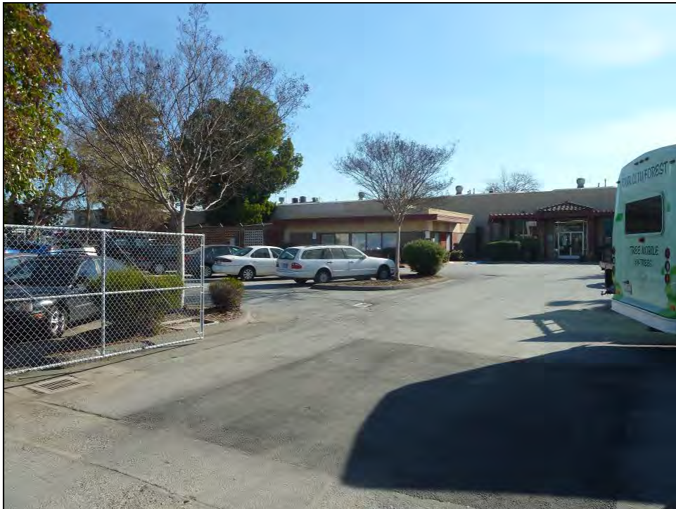
Photograph 2. Showing the 1590 entrance at right of frame and small addition in center, camera facing southeast, January 14, 2015.
