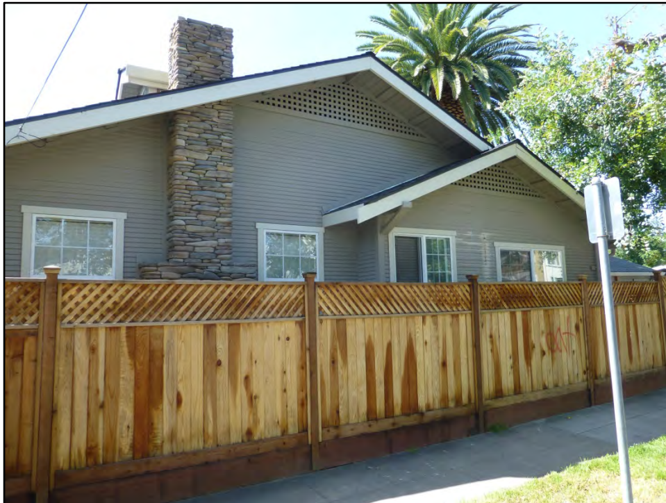
Photograph 2: North side; facing southwest, April 20, 2016.
