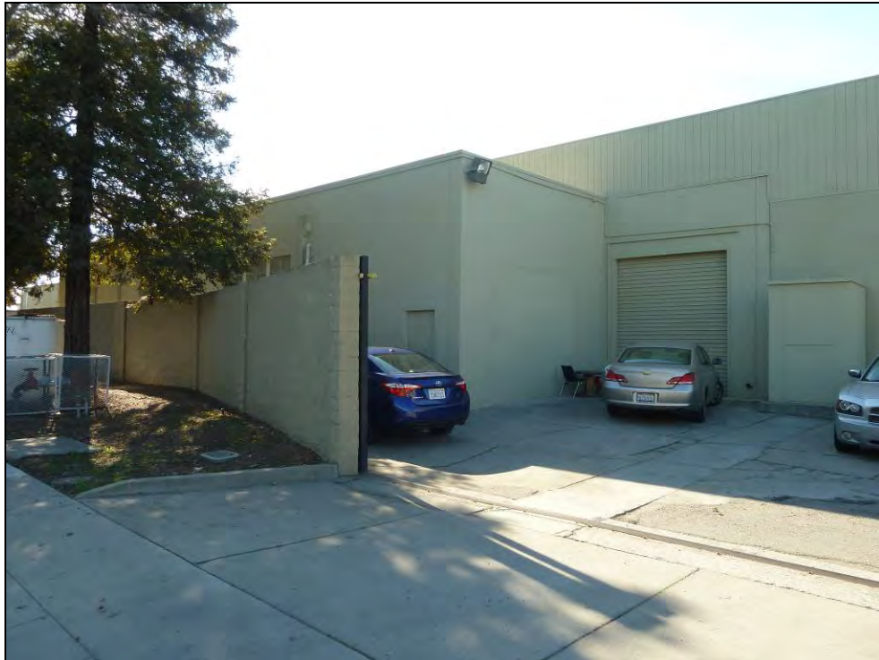
Photograph 4. Section D on left and Section J on right, camera facing southwest, January 14, 2015.
