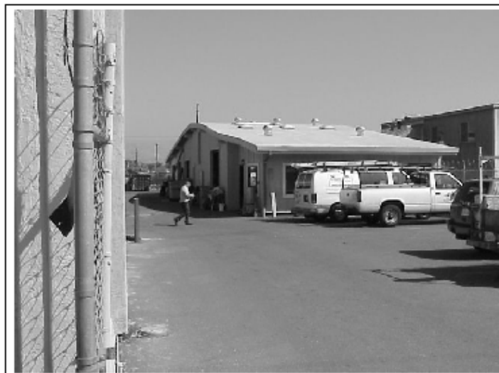
Photograph 2: 610 Stockton Avenue, camera facing east, October 4, 2000.
