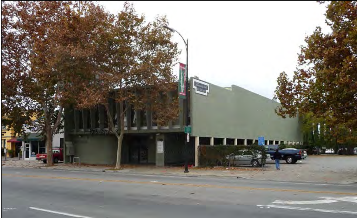
Photograph 1. Camera facing northwest, November 19, 2013
