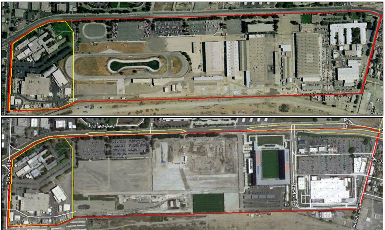
Figure 1. Aerial views of the FMC Corporation facility in 2002 (top) and 2016 (bottom) showing historical parcel boundary in red and parcel boundary for APN 230-46-069, which is documented on this form, shown in yellow at left. The buildings on the subject parcel were under active demolition at the time of the present survey. 3
