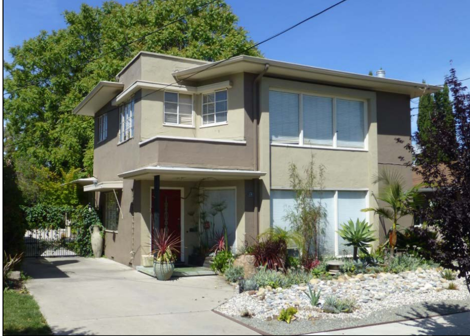
Plate 19. Mid-Century Modern duplex at 179-181 Rhodes Court, San Jose (Map Reference # F-2). (Photograph by JRP)
