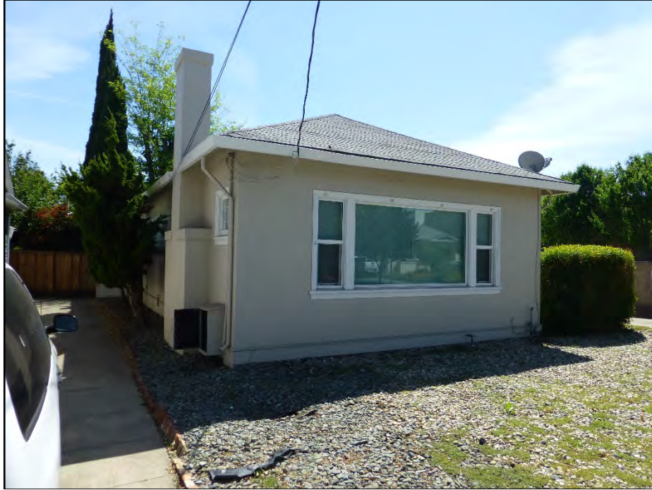
Photograph 2: 128 Rhodes Court, camera facing southeast, April 20, 2016.
