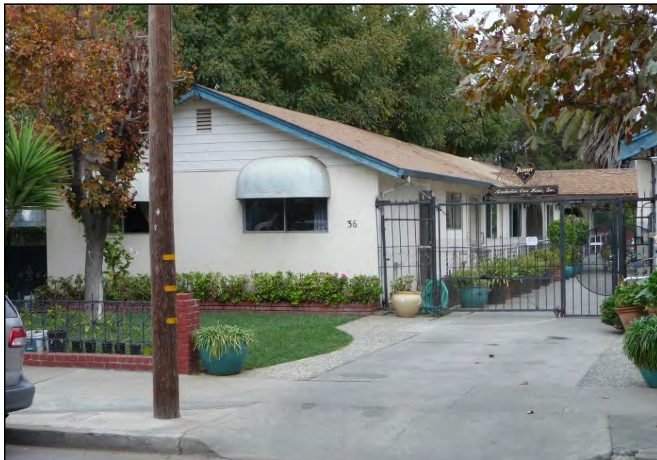
Photograph 3: North building and connecting breezeway, camera facing northeast, November 19, 2013.
