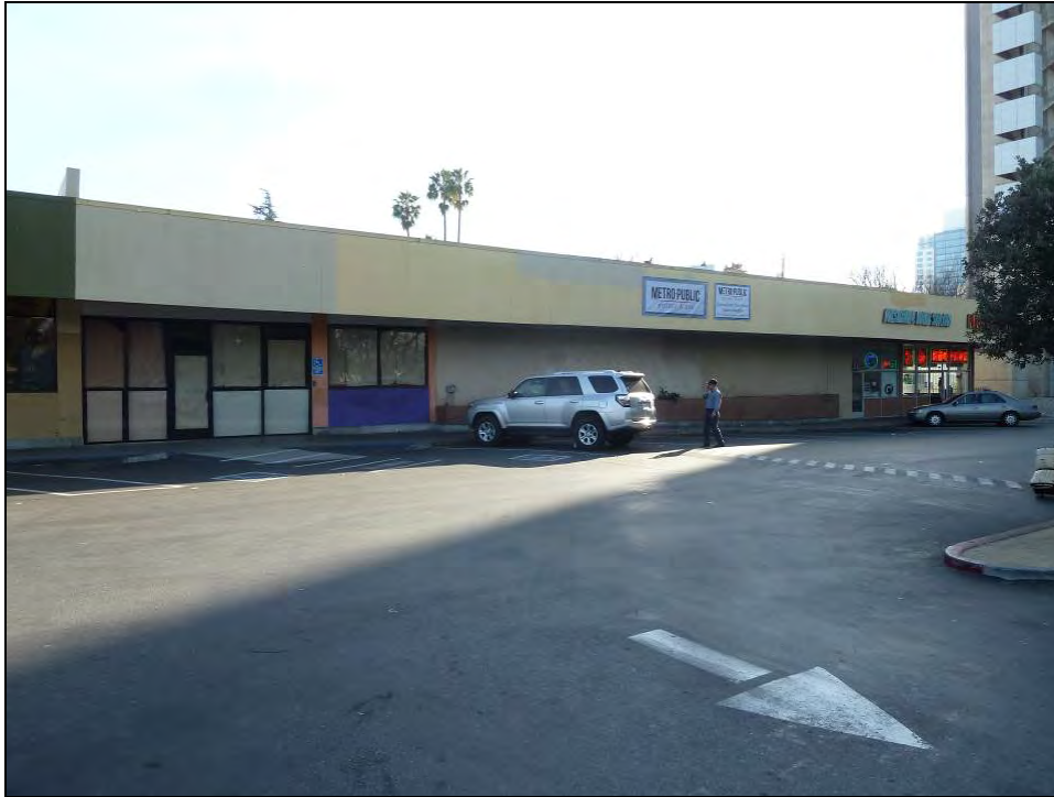
Photograph 3. West half of building, camera facing southwest, January 14, 2015.
