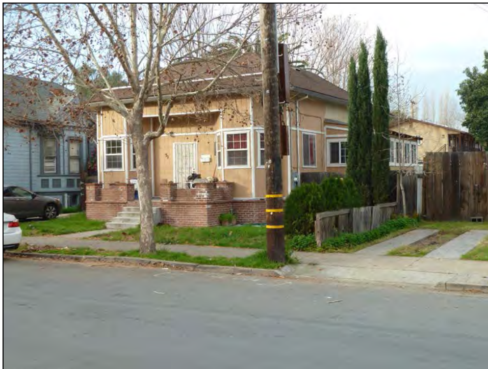
Photograph 2: East and south sides, camera facing northwest, January 16, 2015.
