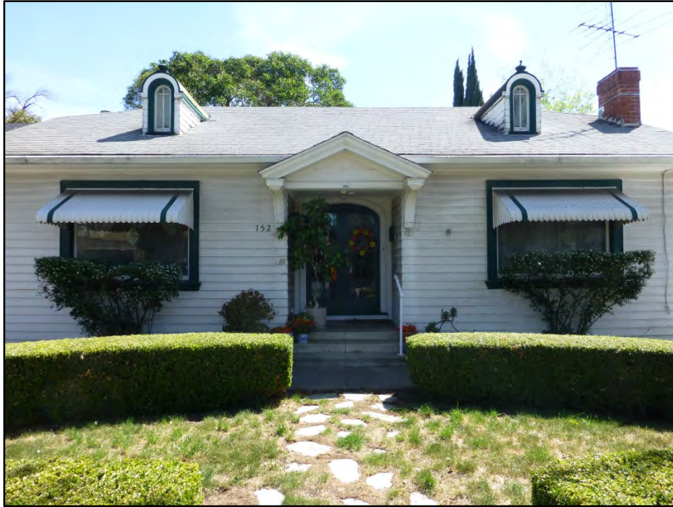
Photograph 2: Main facade; facing east, April 20, 2016.
