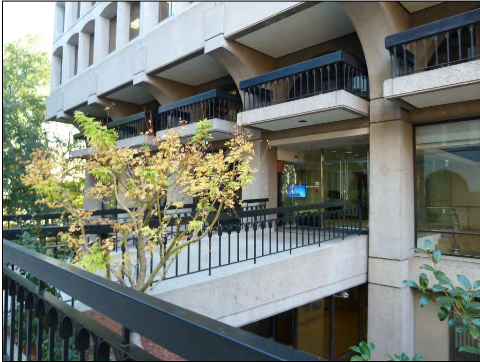
Photograph 4: North entrance, camera facing southeast, December 5, 2013.
