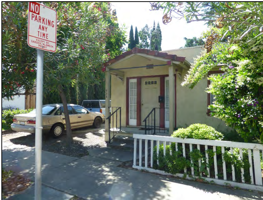
Photograph 2: 936 West Julian Street, camera facing southeast, April 20, 2016.
