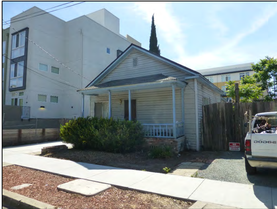
Photograph 2: 850 Cinnabar Street, camera facing southwest, April 20, 2016.
