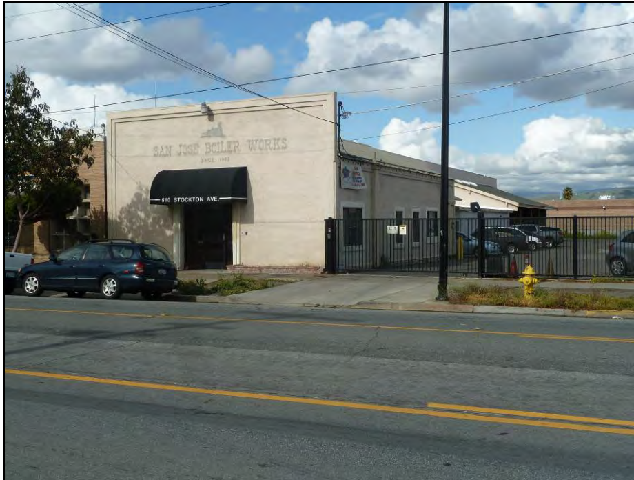
Photograph 1: San Jose Boiler Works, camera facing east, March 26, 2014.
