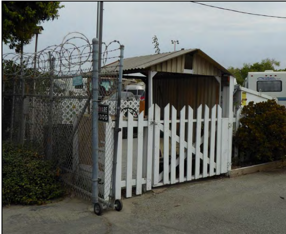
Photograph 4. Storage shed, camera facing northeast, September 14, 2015.
