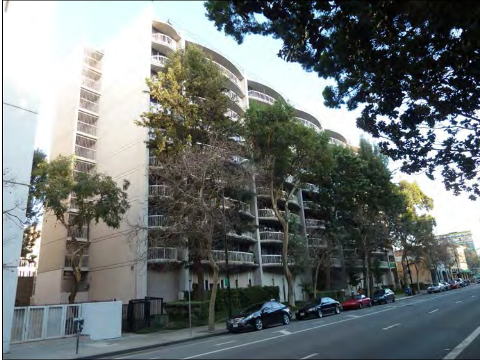
Photograph 2. Building façade, camera facing southeast, January 14, 2015.
