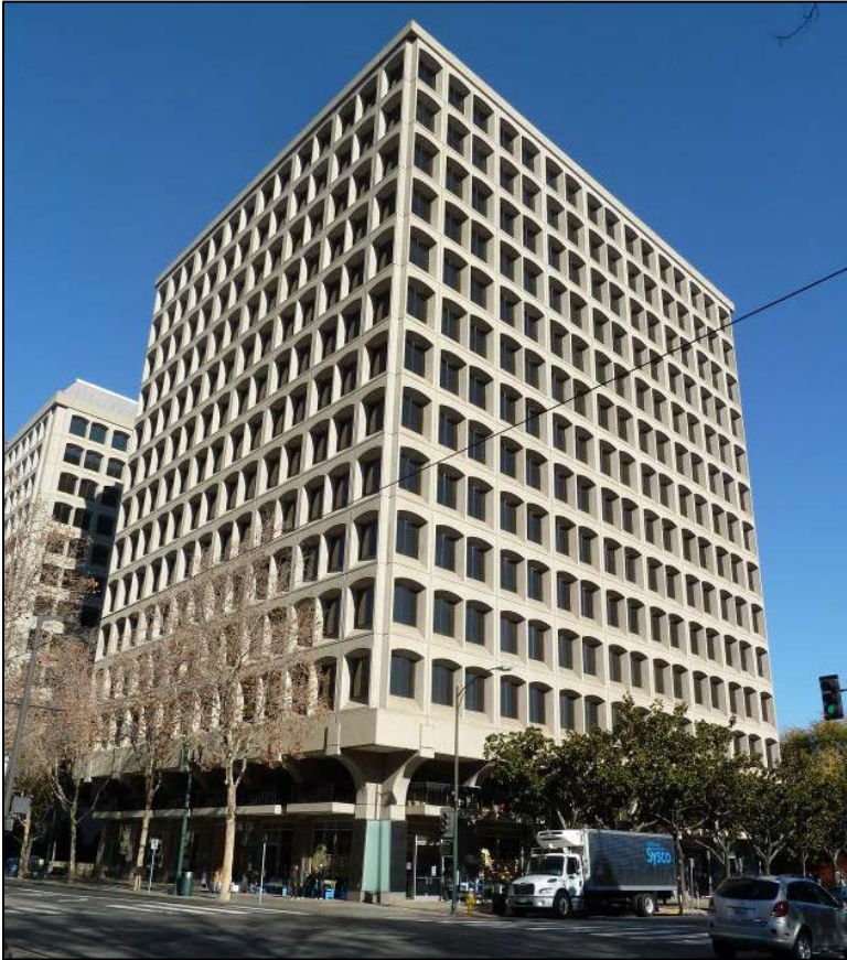
Plate 14. Commercial Modern with Brutalist Influences, 1970s, at 2 N. 2 nd Street (Map Reference # E-02). (Photograph by JRP)
