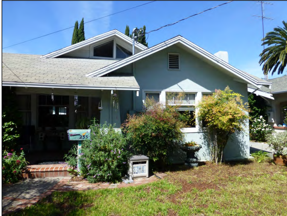
Photograph 2: Front porch with tapered columns; facing west, April 20, 2016.
