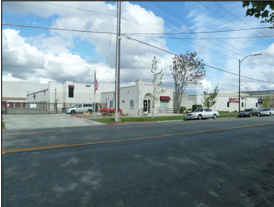
Photograph 1. 580 Stockton Avenue showing the 1925 building in center of photo, camera facing southeast, March 26, 2014.
