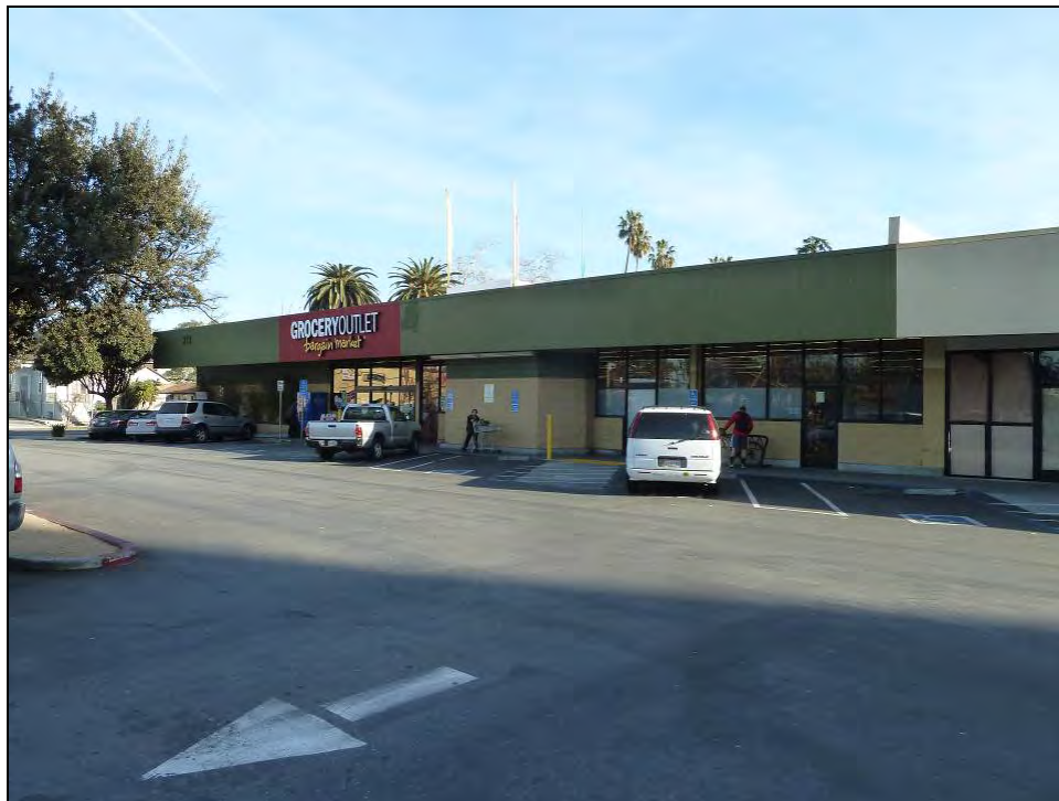
Photograph 2. East half of building, camera facing southeast, January 14, 2015.
