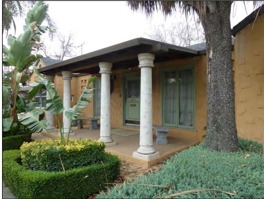
Photograph 2: Detail of east entry, camera facing south, January 16, 2015.
