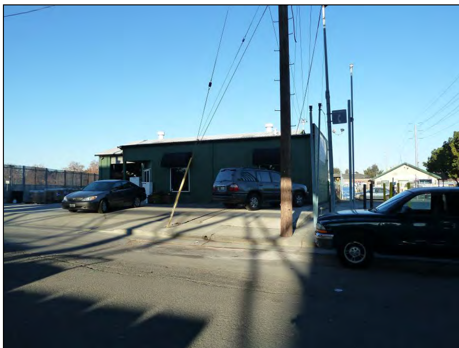
Photograph 2: Showing south side of 1963 addition, camera facing north, December 5, 2013.
