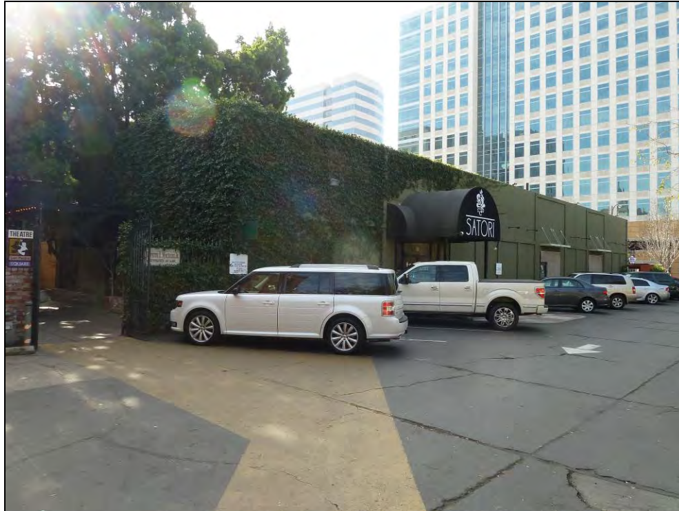
Photograph 2. North side of building, camera facing southwest, January 15, 2015.
