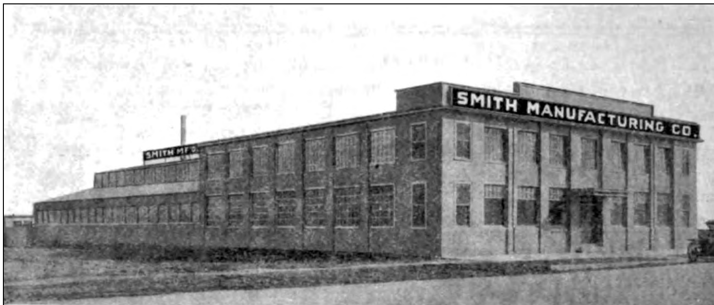
Illustration 1: Smith Manufacturing Company building, as it appeared when it opened in 1917. 6
