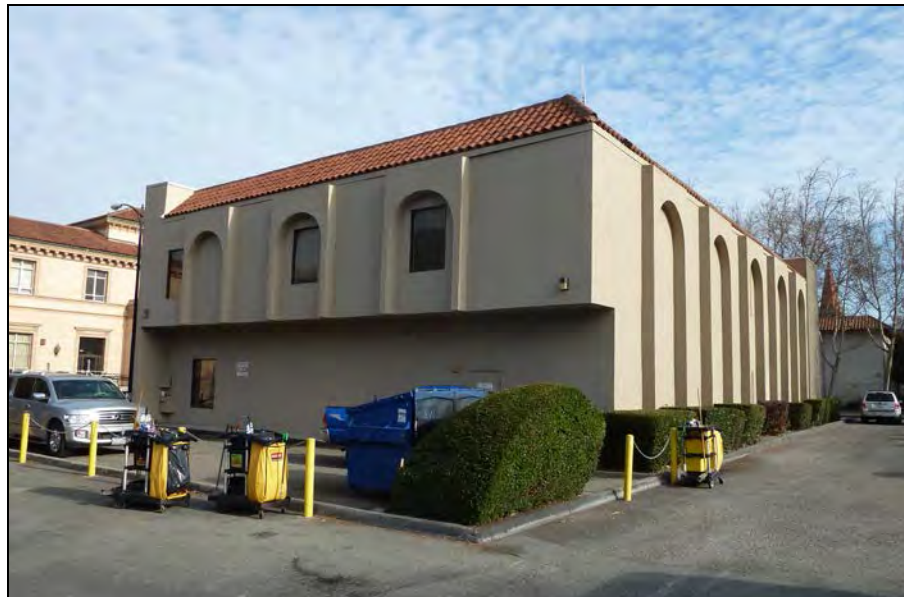
Photograph 2: West and south sides, facing northeast, January 15, 2015.
