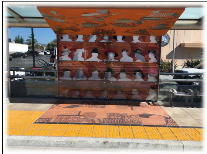
BRT Station shelter - Jackson St Eastbound Station
