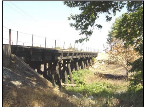
Llagas Creek Bridge
