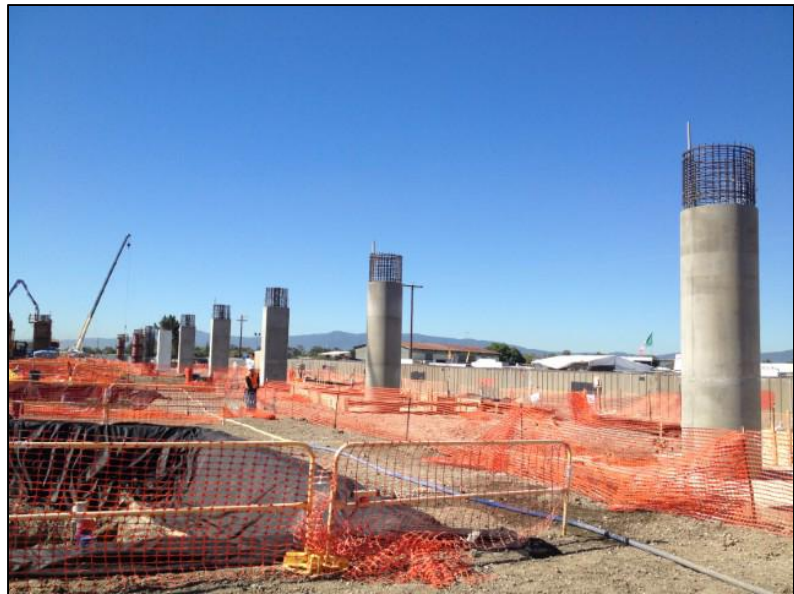
Berryessa Aerial Structure Columns (C700)
