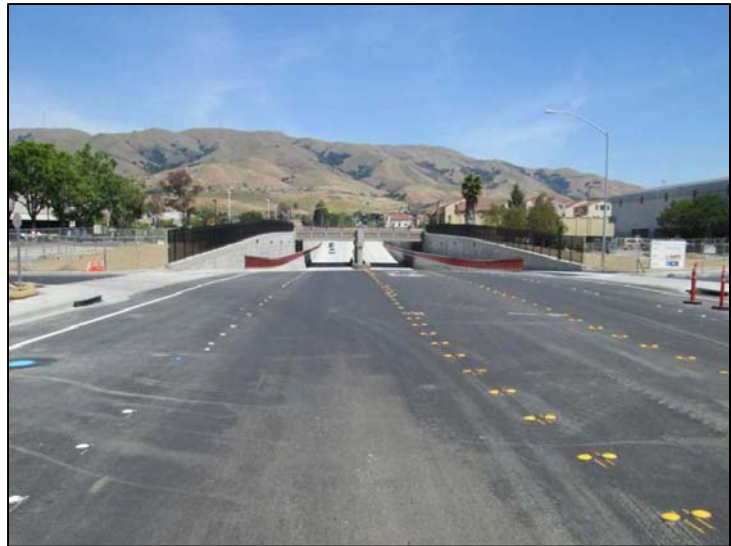
Kato Road open to traffic
