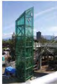
Elevator at the Hamilton Light Rail Station
