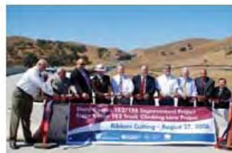
Newly opened SR 152/156 flyover provides increased safety and congestion relief
