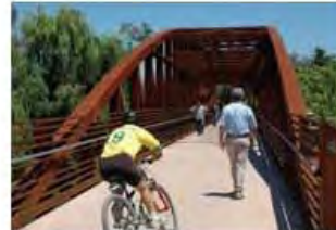
River Oaks Bicycle/Pedestrian Bridge
