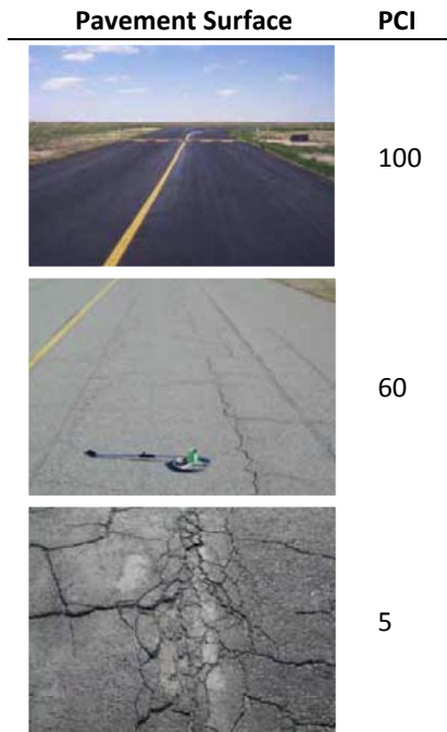
Figure 4 Example Pavement Surface & PCI
