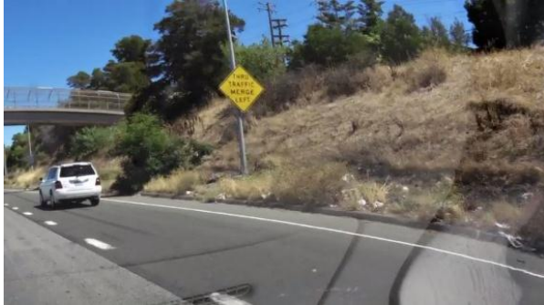
I-680 NB Before McKee Rd
