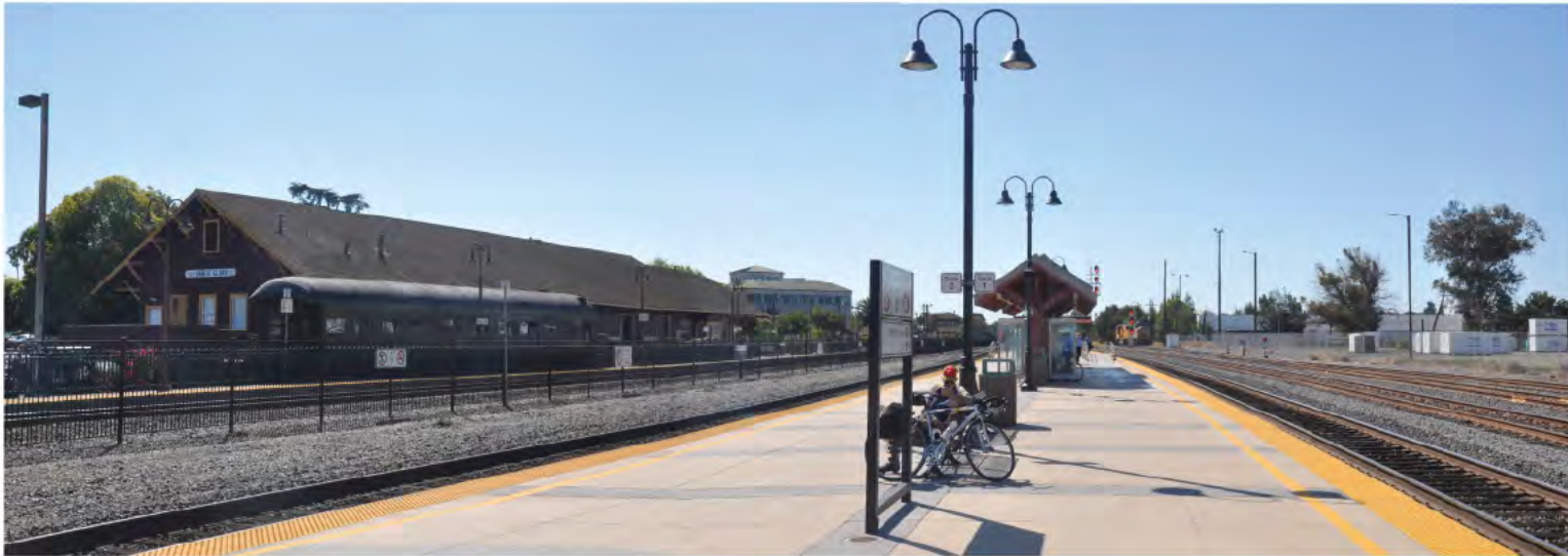
Existing view of the Santa Clara Caltrain Station and Platform (view to the northwest from the Santa Clara Caltrain Station platform)
