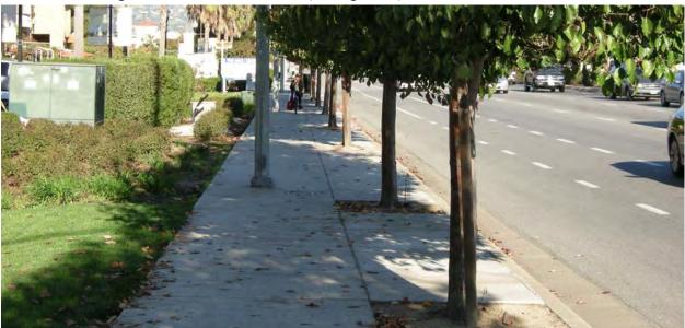
Figure 17: Placement of roadway light fixtures along the back of sidewalk requires wheel chair users to meander around light fixtures and tree locations
