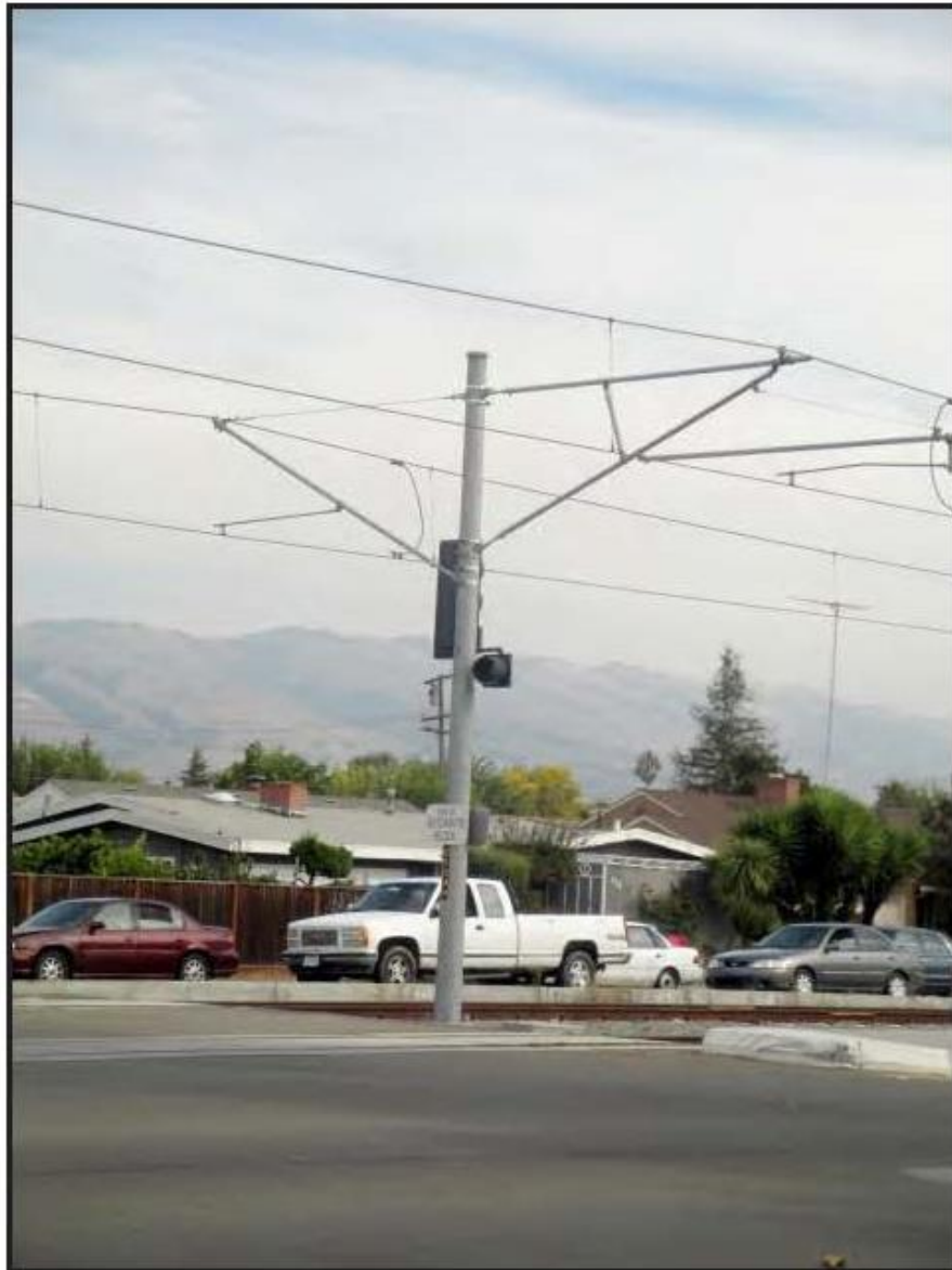
Figure 4 Overhead Contact System at Alum Rock Station
