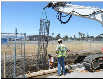
Pile foundation for platform at Ocala Bus Station
