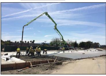
Concrete pour on the north section of the new loop road
