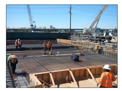
Deck Reinforcing Steel Installation at Montague Overhead Structure
