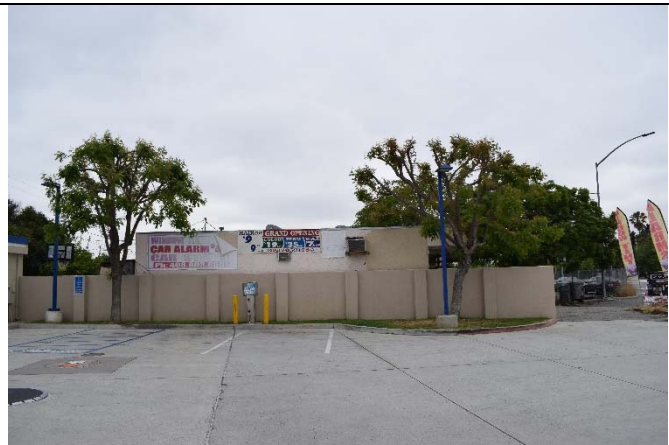
Figure 4. View of south façade, facing north, 5/22/2018.
