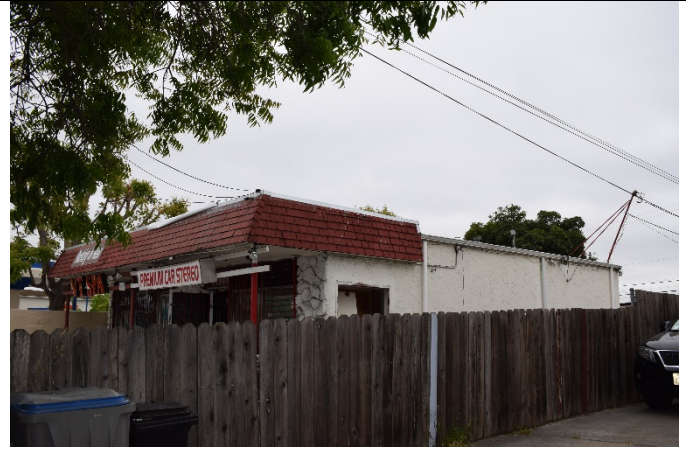
Figure 3. View of north façade, facing south, 5/22/2018.
