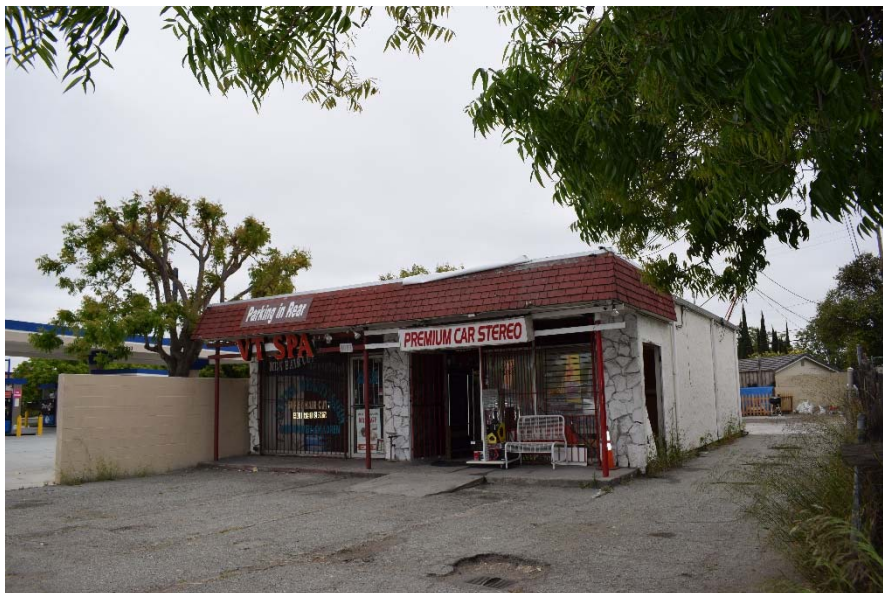
Figure 1: View of east (primary) façade, facing west. Source: ICF.
