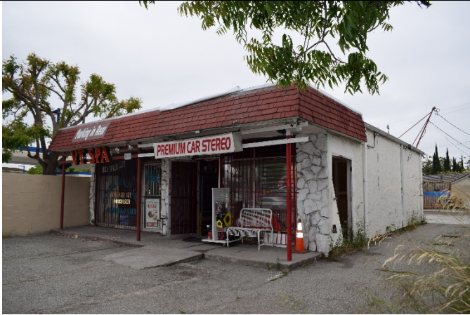
Figure 2. View of east façade, facing west, 5/22/2018.
