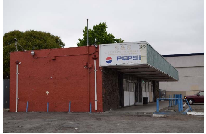
Figure 3. View of west façade, facing east, 5/22/2018.
