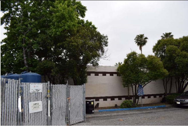
Figure 4. View of north façade, facing south, 5/22/2018.
