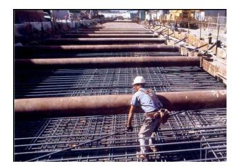
Figure 4.19-15: Installation of Station Roof
