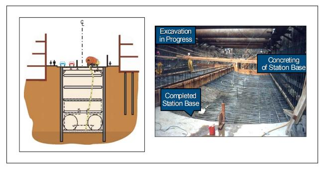
Figure 4.19-14: Installation of Base Slab
