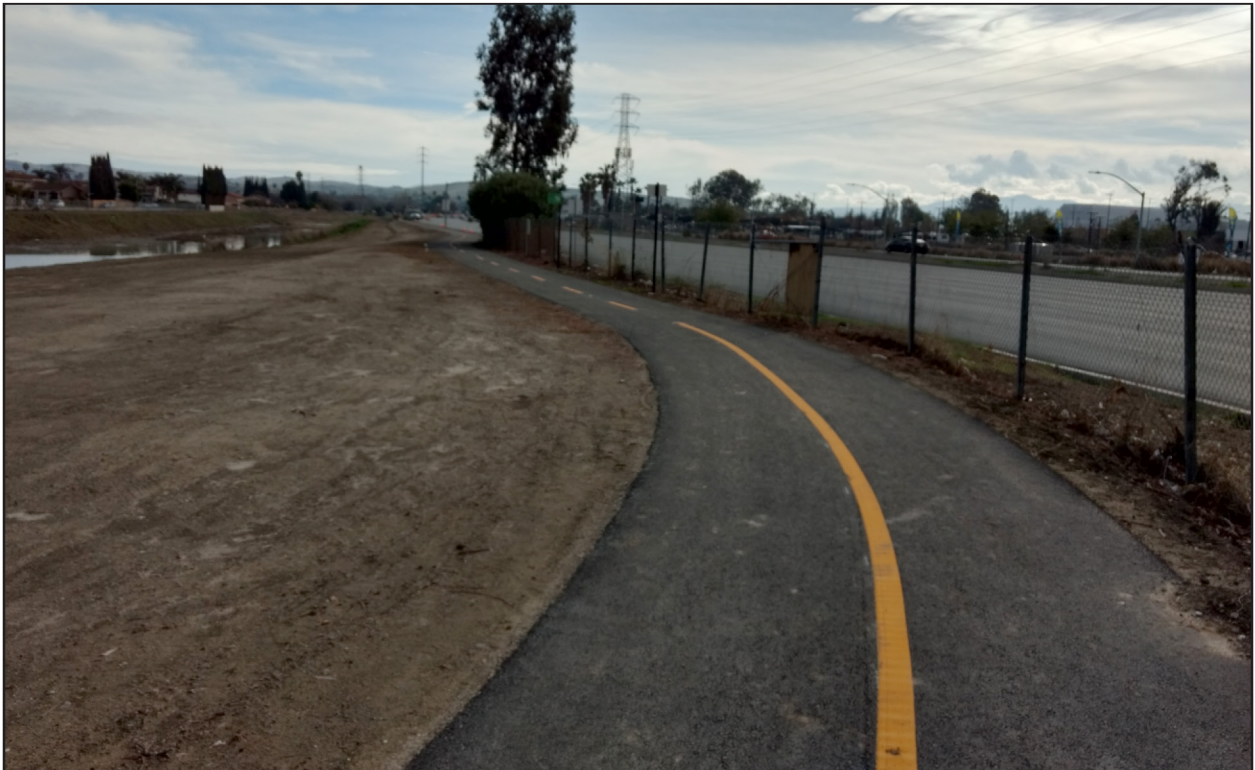
b. View of trail facing south toward the intersection of Capitol Expressway and Capitol Expressway Connector Road at Eastridge Mall.
