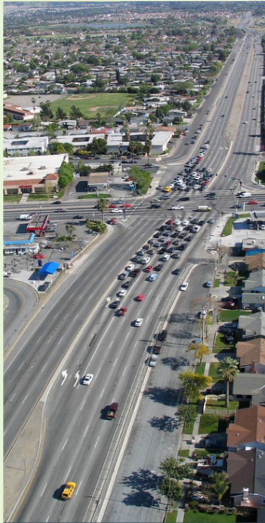
Existing Story Road
