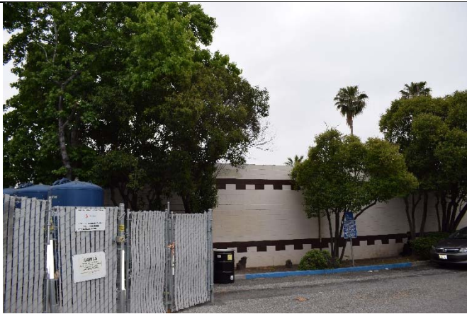
Figure 4. View of north façade, facing south, 5/22/2018.
