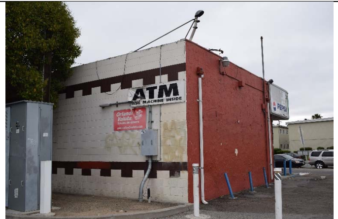
Figure 5. View of north and west façade, facing southeast, 5/22/2018.
