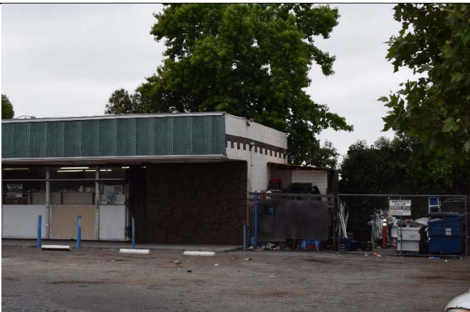
Figure 6. View of east facade, facing north, 5/22/2018.
