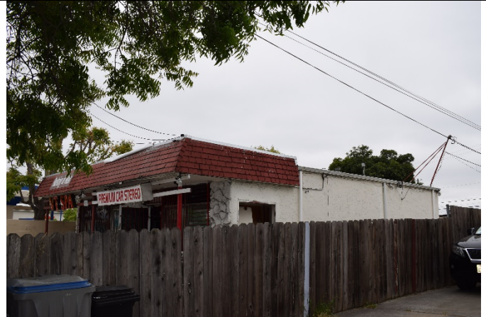
Figure 3. View of north façade, facing south, 5/22/2018.
