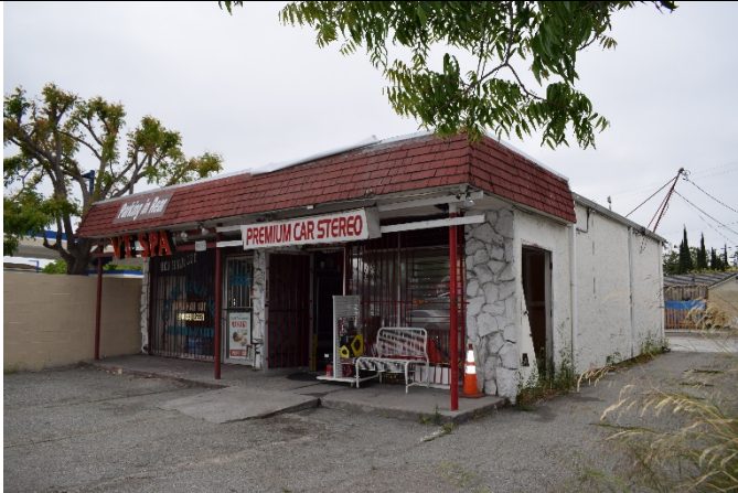
Figure 2. View of east façade, facing west, 5/22/2018.
