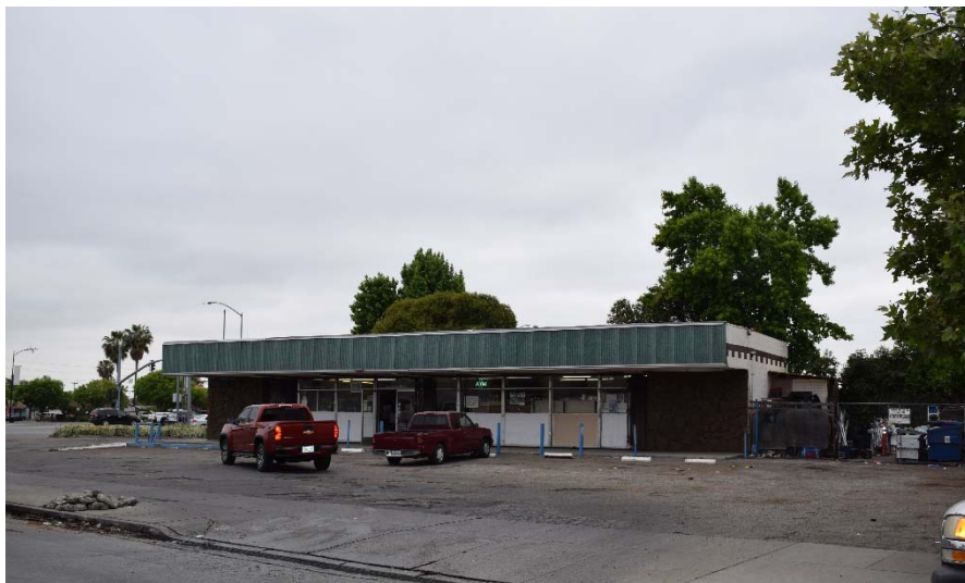
Figure 1: View of south (primary) façade, facing north. Source: ICF.
