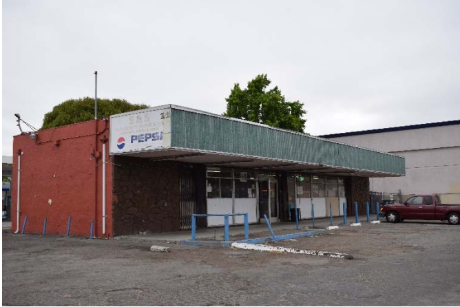
Figure 2. View of south façade, facing northeast, 5/22/2018.
