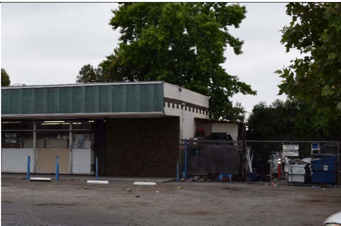
Figure 6. View of east facade, facing north, 5/22/2018.
