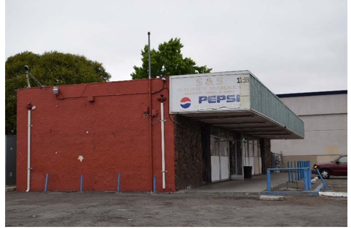
Figure 3. View of west façade, facing east, 5/22/2018.
