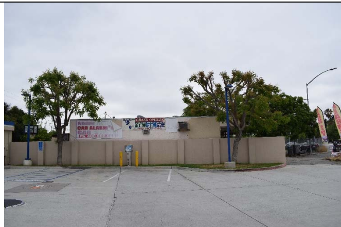
Figure 4. View of south façade, facing north, 5/22/2018.
