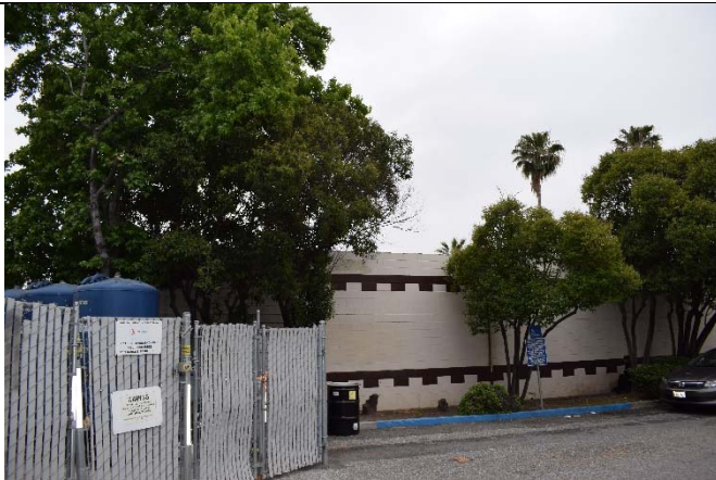
Figure 4. View of north façade, facing south, 5/22/2018.
