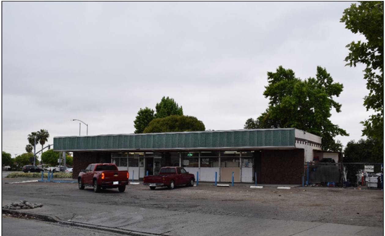
b. View of the building at 1148 S. Capitol Avenue.
