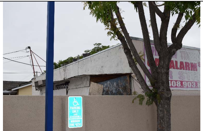
Figure 5. View of west (rear) façade, facing east, 5/22/2018.
