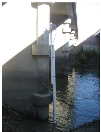
**Photo B-1.** Water-level datasonde installed during a low tide on the Guadalupe River.
