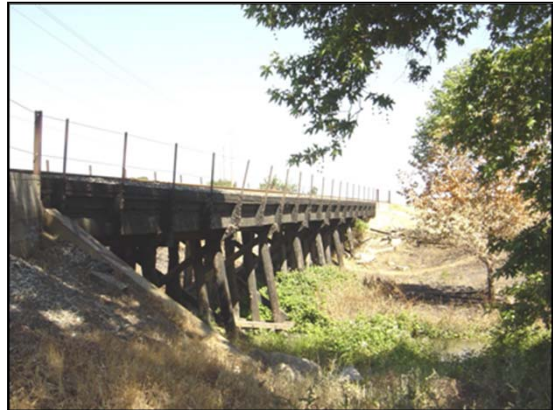
Llagas Creek Bridge
