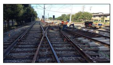
Turnout and switch machine installation in progress near Stevens Creek Bridge
