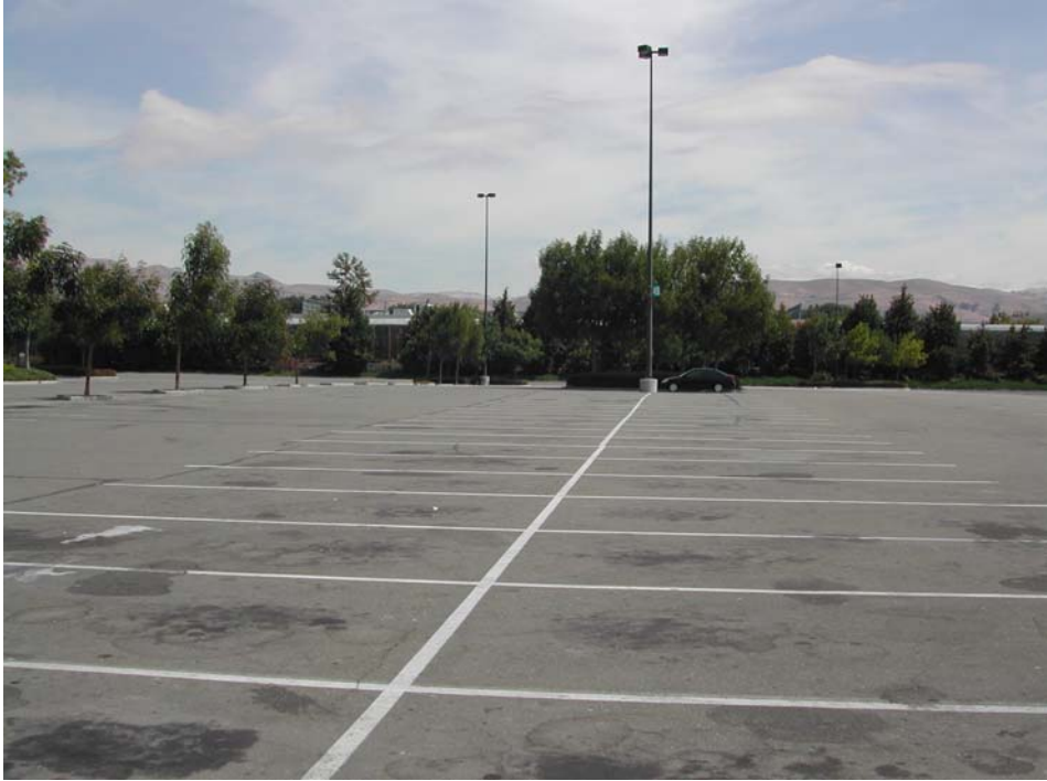
Looking East Toward the Railroad Tracks from the Great Mall Parking Lot
