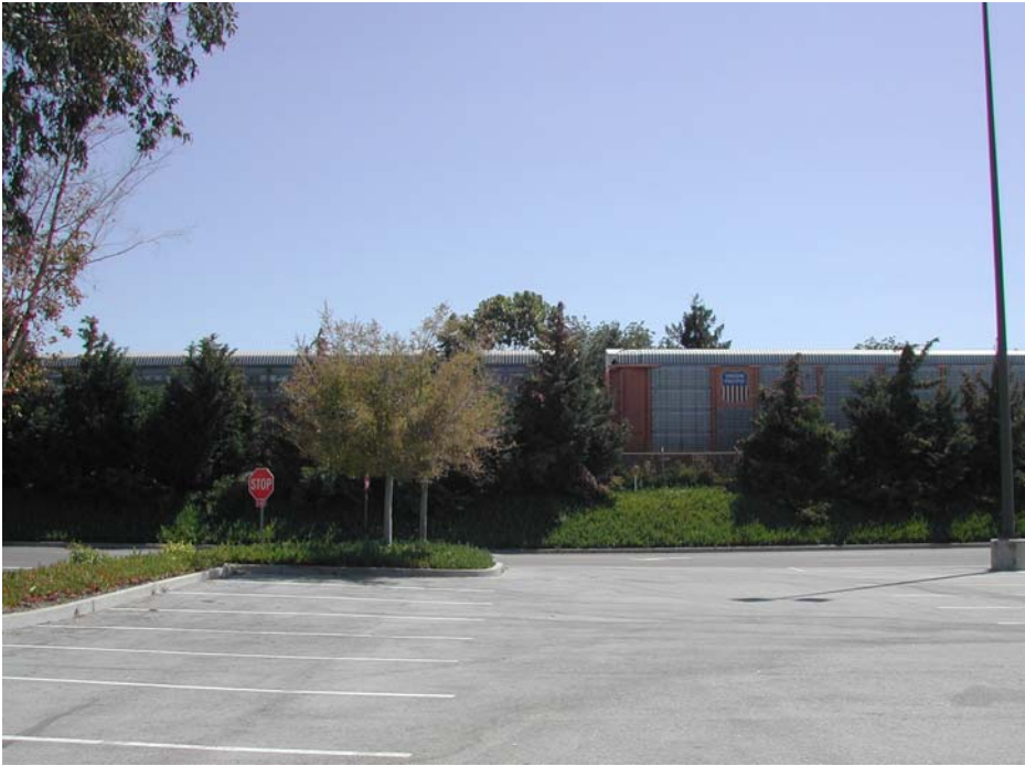
Looking East Toward the Railroad Tracks from the Great Mall Parking Lot
