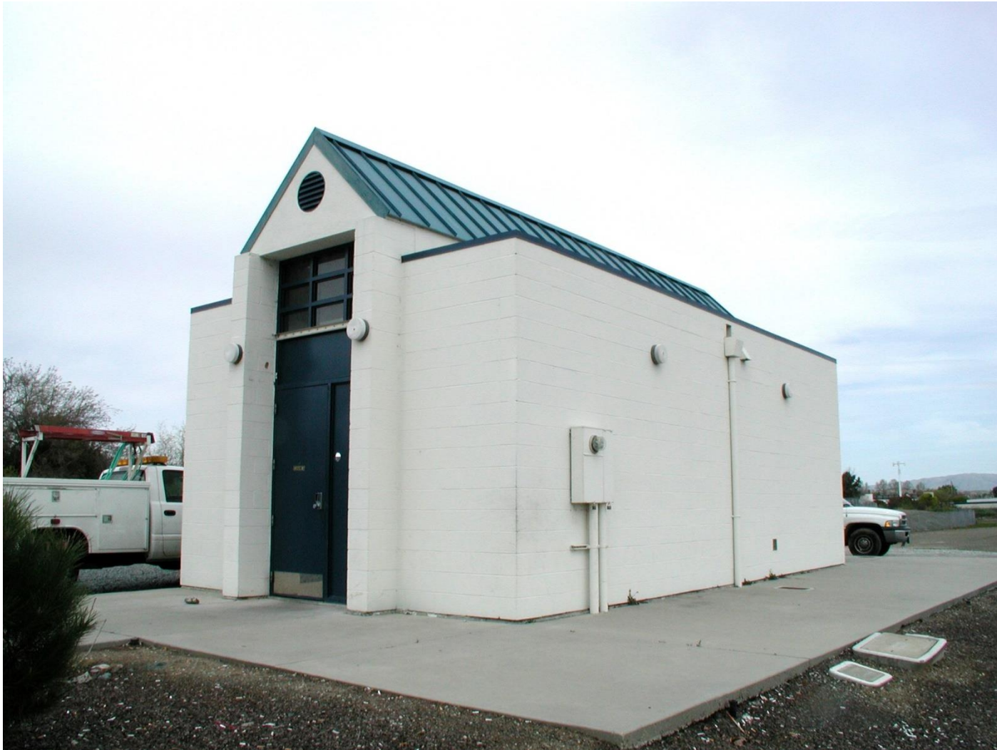
Almaden Operators Break Room
