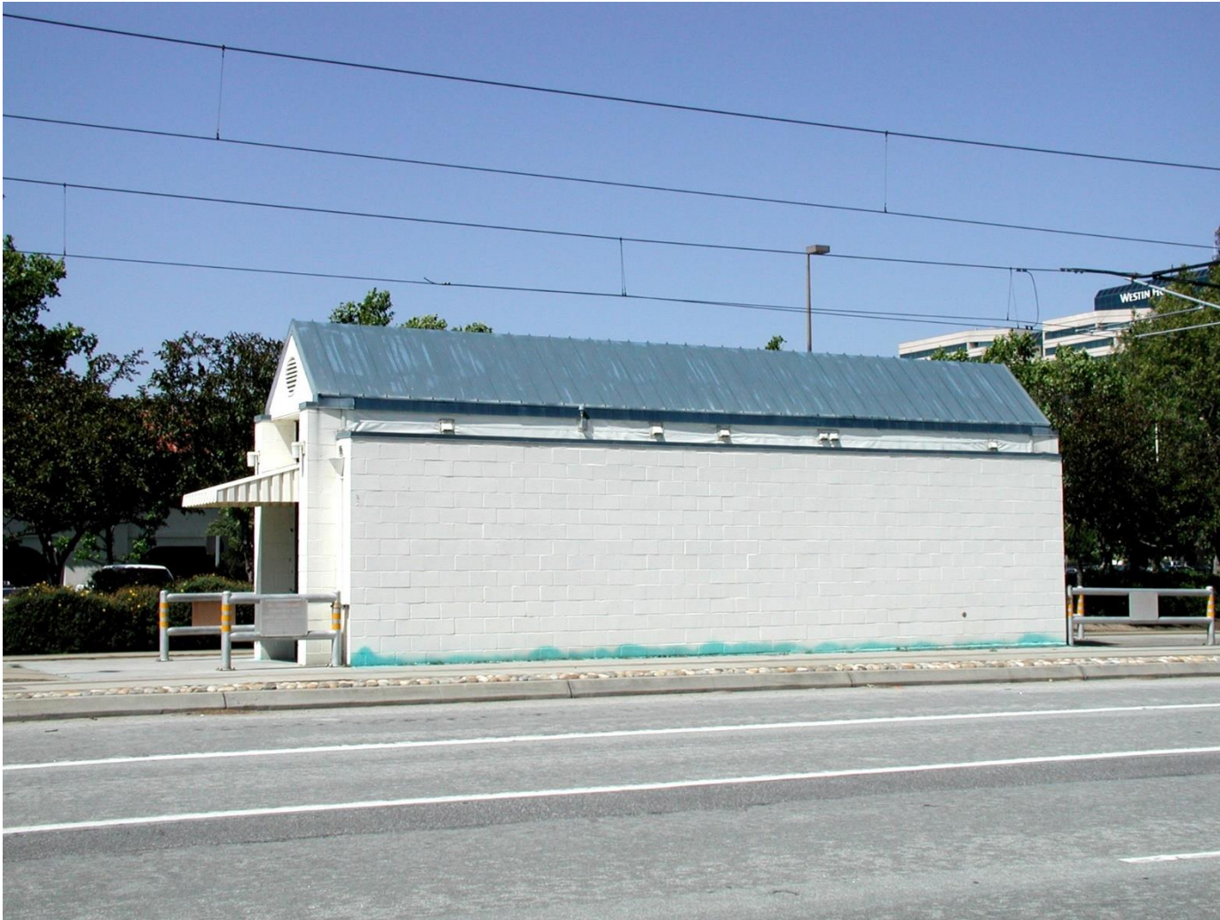
Old Ironsides Operators Break Room
