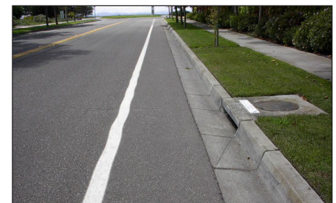
Curb-face inlet on newly built street section in Alameda with access to catch basin provided in the landscape strip.
