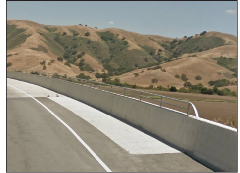
The S.R. 152 flyover of S.R. 156 adds a bicycle railing as it gains elevation. Since bicyclists will only be on the right hand shoulder, it is only needed on the right side of the flyover.
