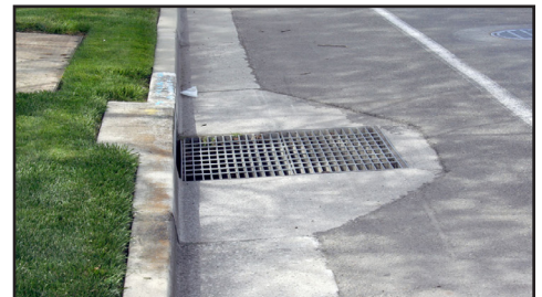
Grate wider than gutter pan reduces usable bike lane width to less than the 36 in. min. specified in HDM §301.2.
